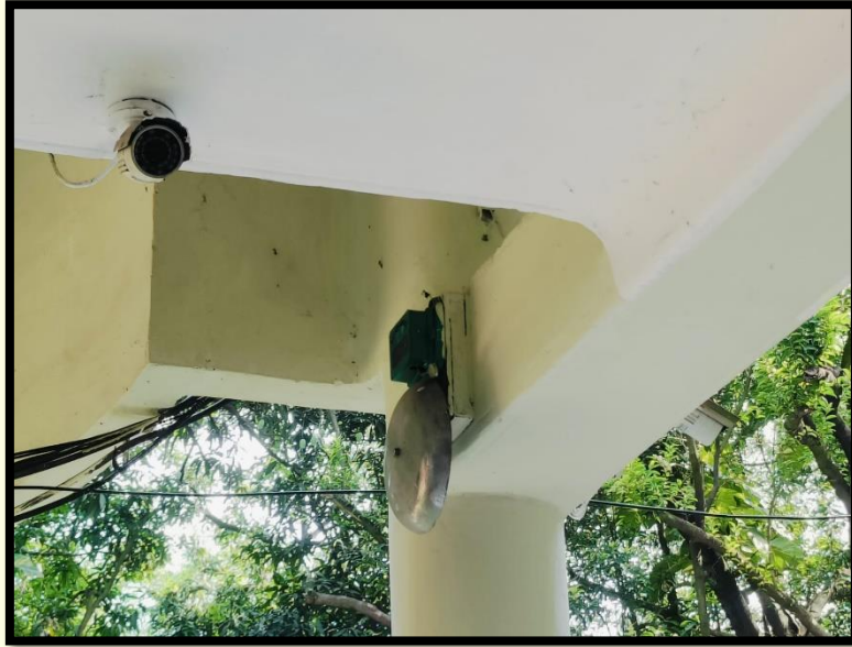
In front of the Principal's Office
