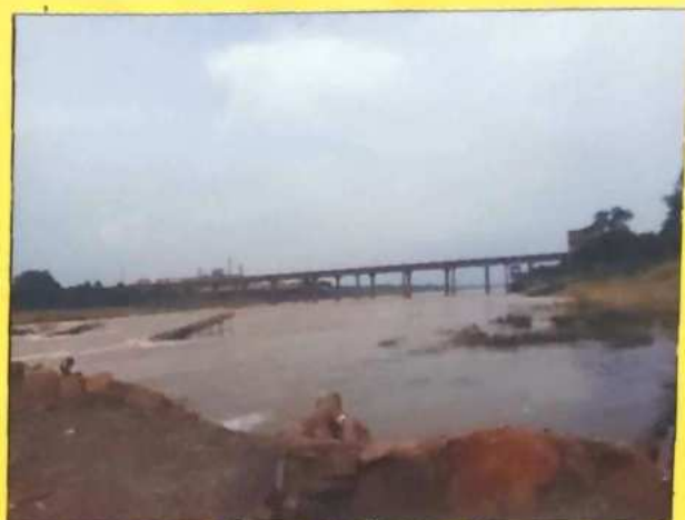
pic.28 DRAINAGE OF TAMAKPAL VILLAGE (SUBARNAREKHA RIVER)
