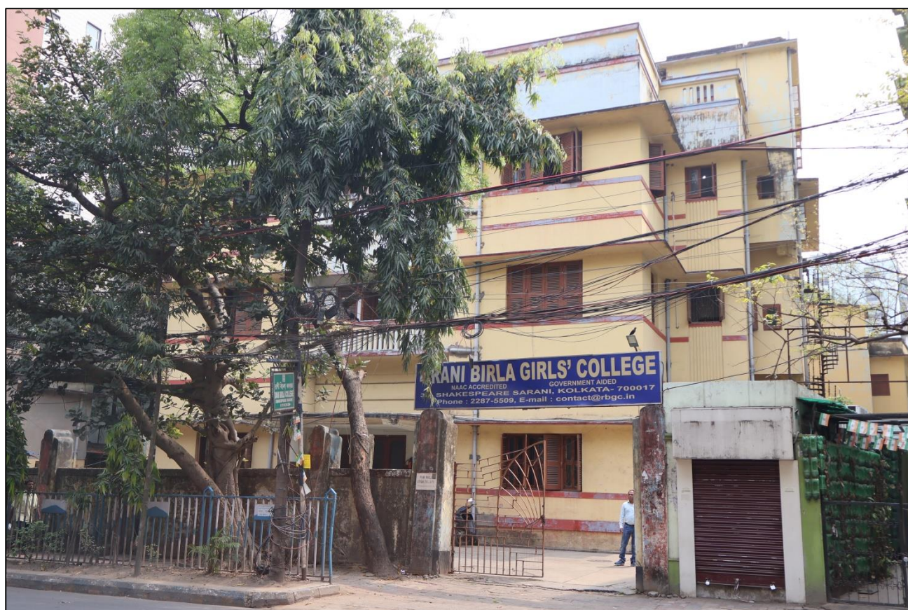
Figure 1: Front view of the College from Main Road side
