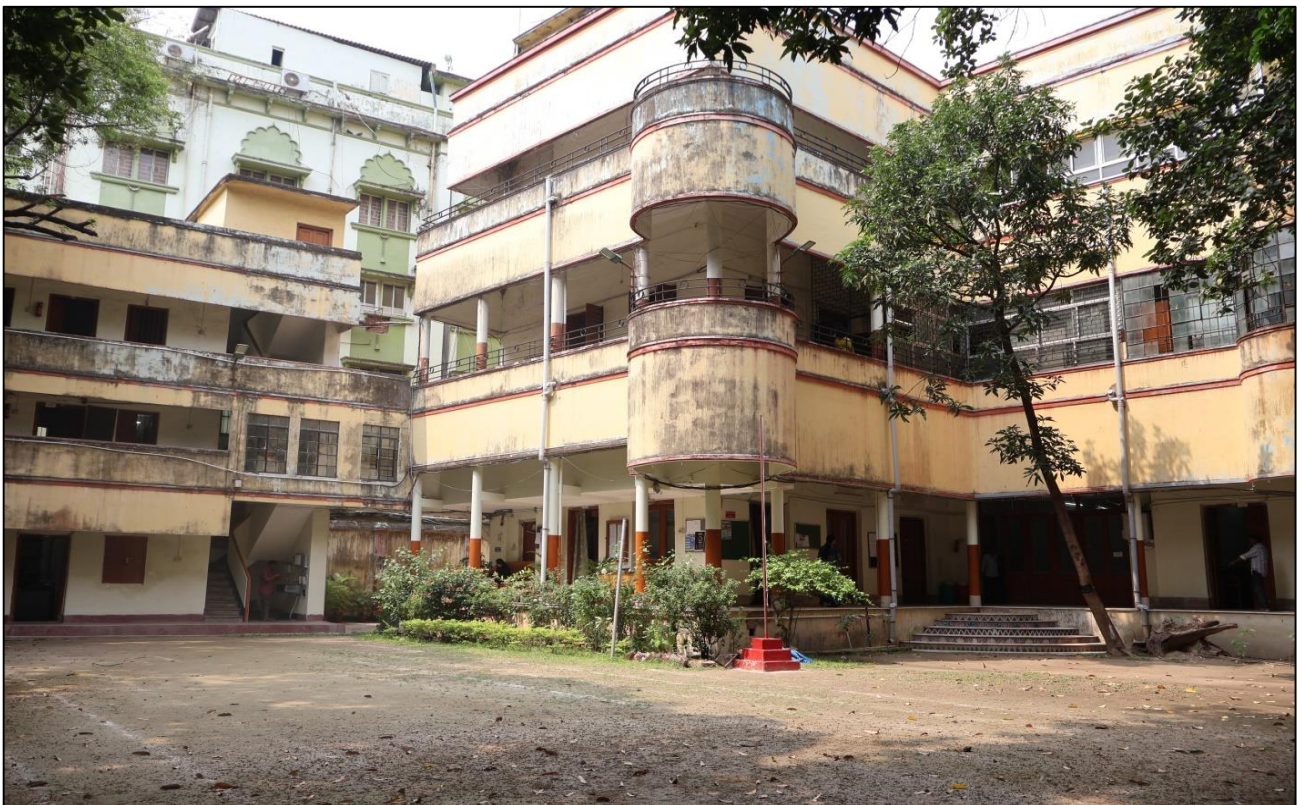
Figure 5: Front and back side view of the College building
