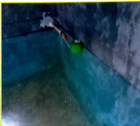
Installed Stop-watch in Water tank to prevent water wastage
