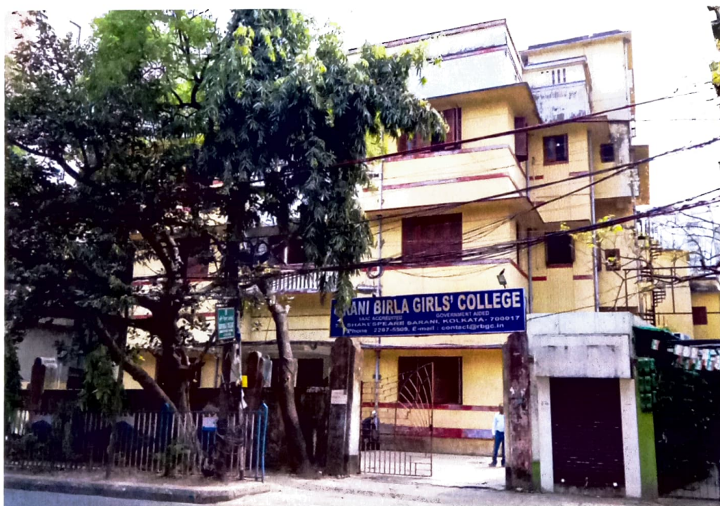
Figure 1: Front view of the College from Main Road side
