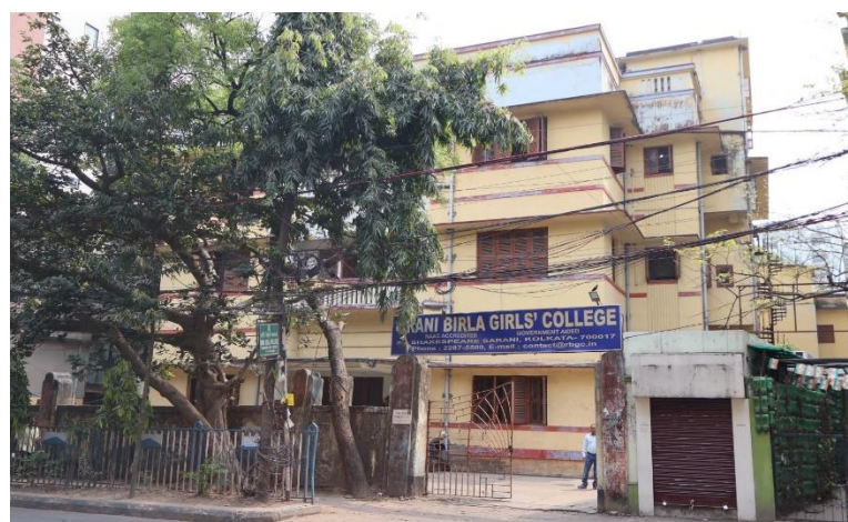
Figure 1: Front view of the College from Main Road side
